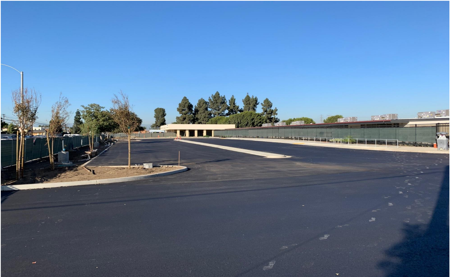
39 Student Drop-off along Dale Ave. (Increment I- Modernization) – Under Construction
