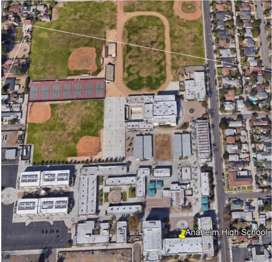
Measure H funding will be used to fund the security fencing. This project is a component of the Anaheim High School Aquatics Center Project.
