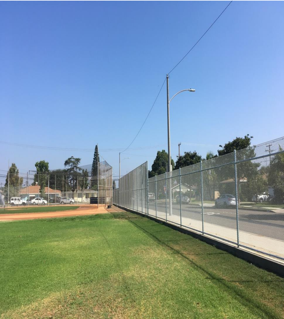
Perimeter Fencing along Sycamore Street
